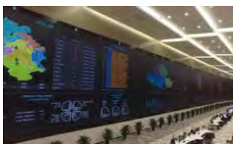
The world's largest video wall with 324 LED DLP 80" cubes and DVCS system in China
